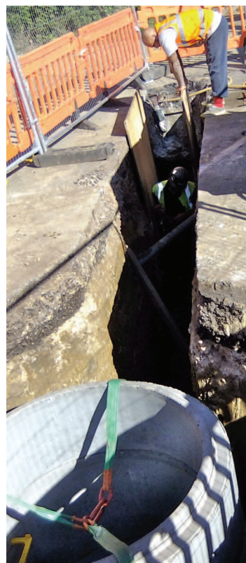
Installation of an inspection chamber for surface water drainage in Ipswich Road, Grundisburgh, part of the major work which has led to its temporary closure.
