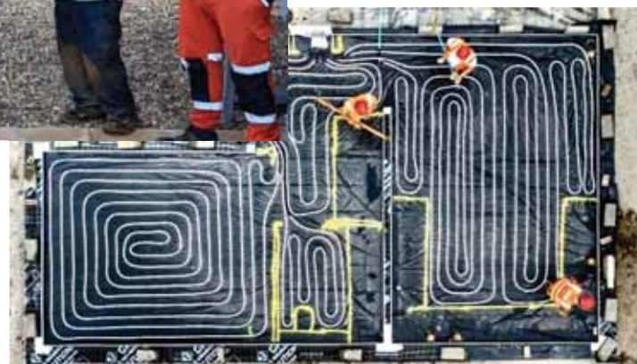
Top: Health and Safety briefing. Above: aerial photo showing team laying underfloor heating on new build houses.
