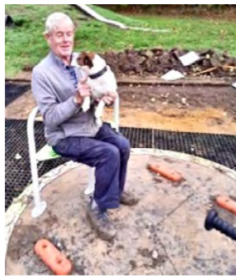
David Lugo (accompanied by Bosun) taking a break from installing the new accessible roundabout. Photo by Jim Bird
