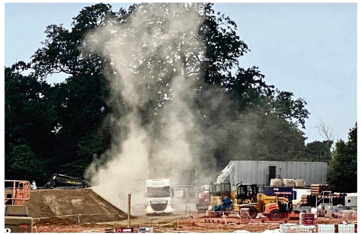
Contractors moving earth from the Chapel Field building site.
